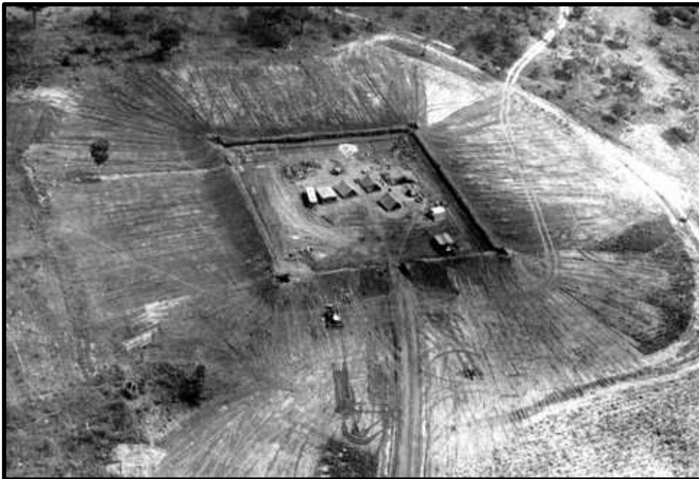
Graphic image of a Bulldozer forming the earthen walls of a keep (Ft Misery, Nembire, Mt Darwin) (Gerry van Tonder collection)
