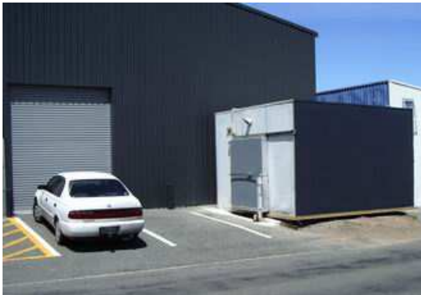
1st top coat on 1 side and the door (28/1/07)
