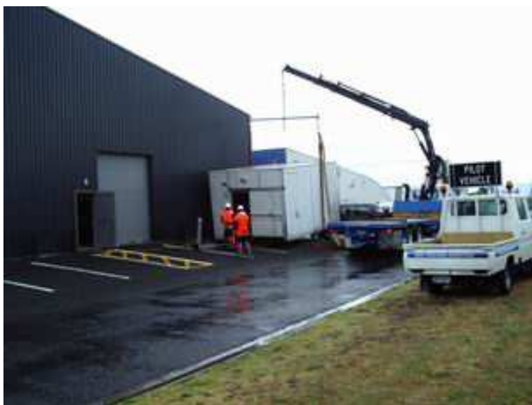
Container shifted in - raining
